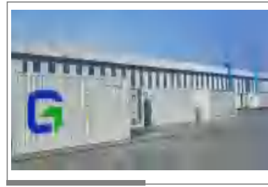
Lithuania ESS Project Scale: 180MWh
